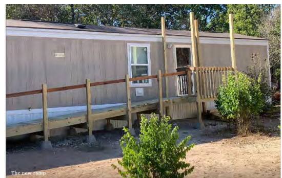
Figure 1:DSHM Featured Project – construction & installation of a new ADA compliant 36 ft long wheelchair ramp
